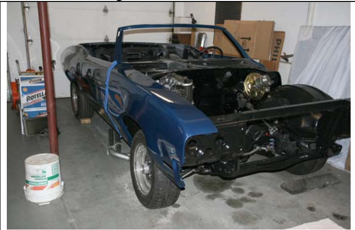
Fitting the new pieces together
